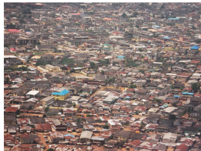
Aerial shot of Lagos, Nigeria, showing the extent of urban sprawl in the city. (Image credit: Sustainable Energy Africa [SEA].)
