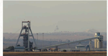
A view of Doornkop Gold Mine, about 30 km west of Johannesburg, South Africa Wednesday, September 4, 2013. A strike by tens of thousands of South African gold miners severely affected production in the struggling industry on Wednesday. There were no reports of violence, and two mining companies reached a settlement with their workers. (AP Photo/Themba Hadebe).
